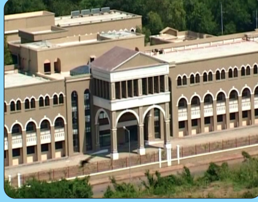
Central Office, HBNI, Mumbai
